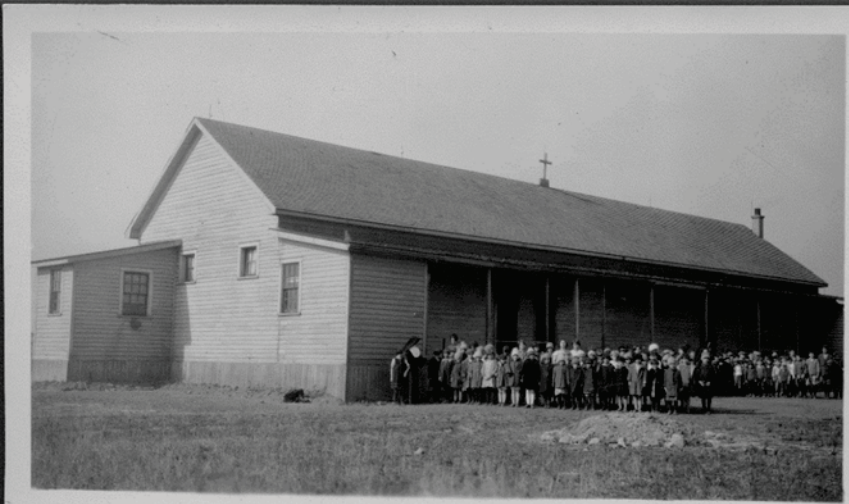
St. Bernard's Bungalow School, Meldrum Road
