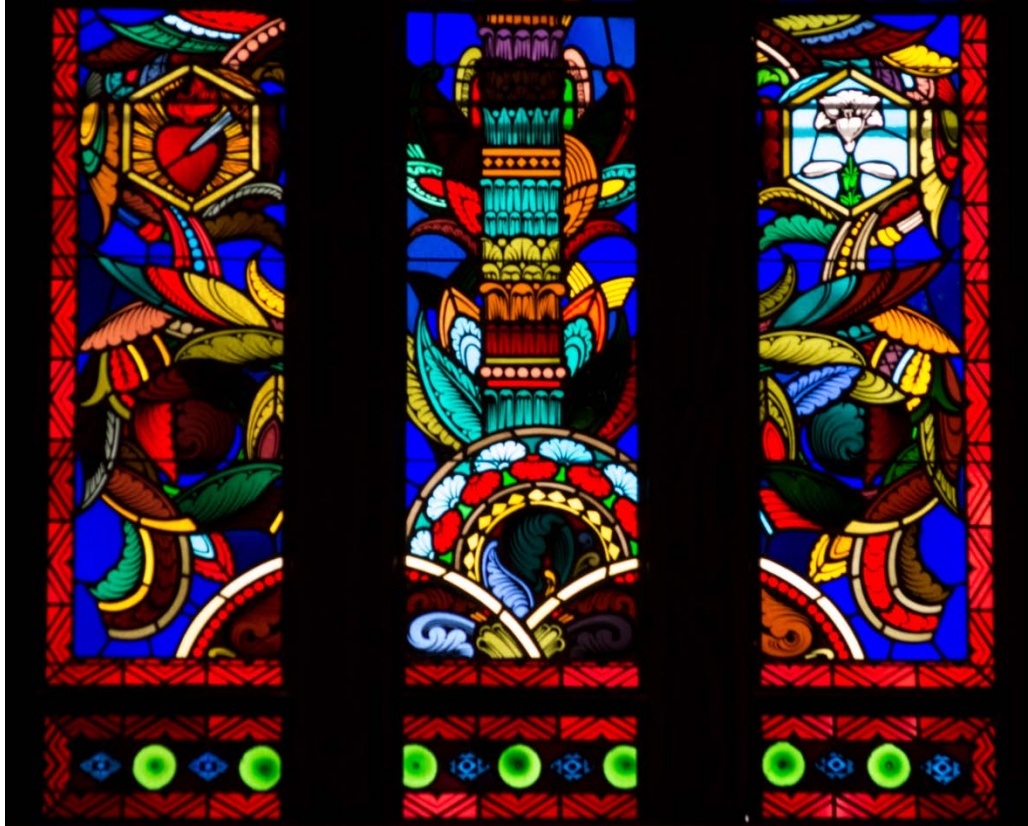
Close-up view of bottom section of southwest sanctuary window
